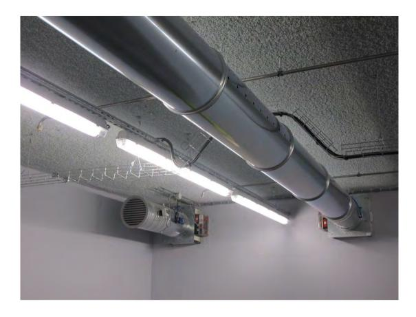
This special air distribution process is sometimes used in the automobile and aeronautical industries when a high level of homogeneity in climatic conditions is desired for large volumes. The air supply duct has perforations calculated to obtain very high induction, ensuring that the ambient air moves with a lower blown airflow rate.
